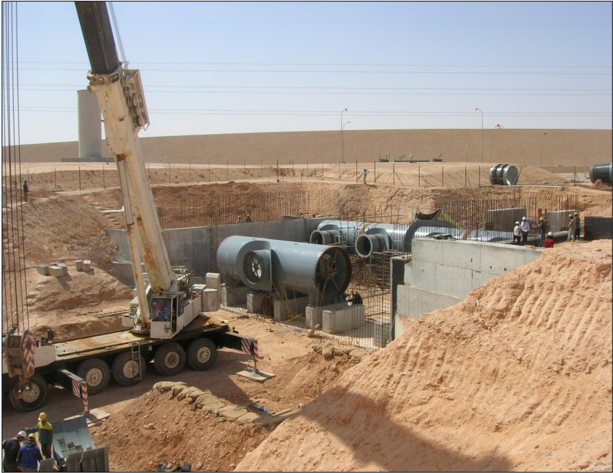
Screen Chamber Construction
