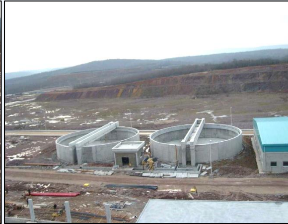
Sludge Thickeners
