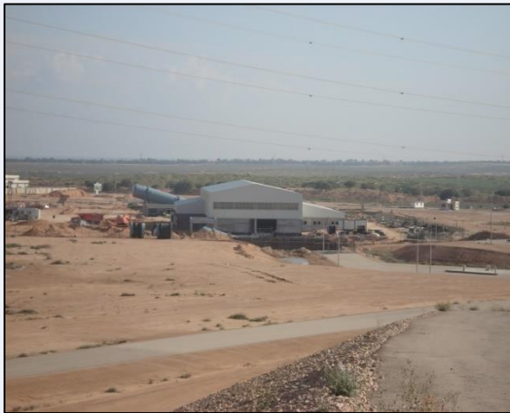
SIRT 'B' Pump Station General View
