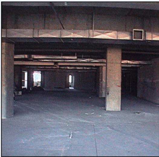
One of the floors before construction started.
